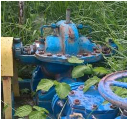
Figure 1 RDN 200-150-200 pump from Doniceasa - Fălcu Plot 7 SPPM (Photo Luca M., 2016)
