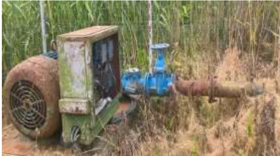
Figure 3 View of 7/5-2 pumping unit (6NDS), electric panel and discharge pipe of the SPPM 7/5 (Photo Luca M., 2016)
