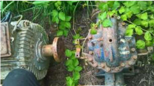
Figure 4 SPPM 7/7-2 pump aggregates status (RDN 200-150-200 pump and motor) (Photo Luca M., 2016)
