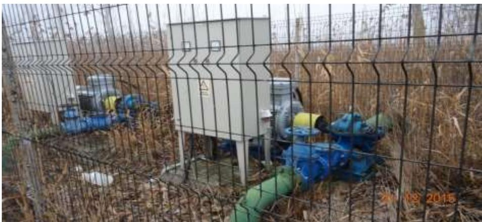
Figure 5 **General view of Doniceasa-Fălcu Plot 7 SPPM SP 7/2, partially rehabilitated (replacement of electric motor and electric panel)** (photo Luca M., 2016)
