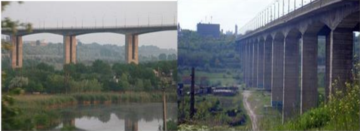
Figure 2 Monitored objective - Viaduct - Galați City, Romania
