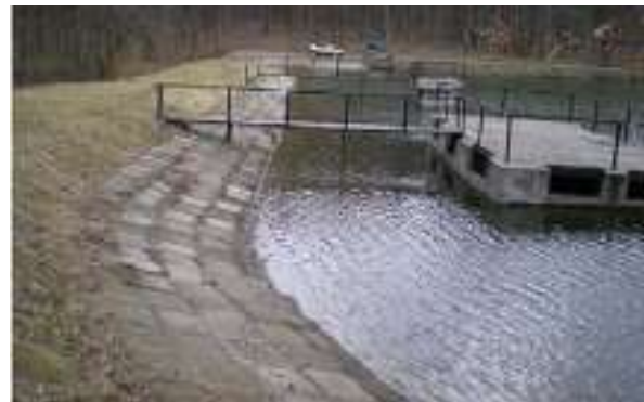
Figure 2 Dam canopy overview - Crujana Dam, Suceava County (ABA Siret, 2010)
