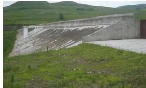
Figure 5 Grănicești Dam, Suceava County, 2008 - general view (ANIF, 2008)
