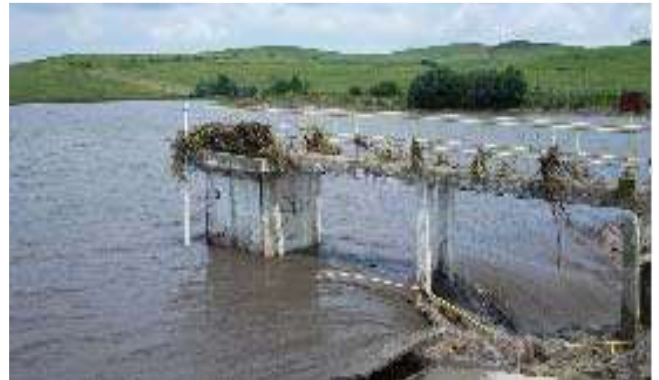
Figure 6 Degradation of the tower at Grănicești Dam, Suceava County, during the 2010 floods (CTM, 2010)
