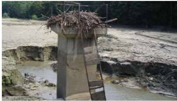
Figure 4 Crujana Dam, Suceava County, 2010 - the maneuvering tower and the lake basin after emptying the lake by breaking the dam (ABA Siret, 2010)
